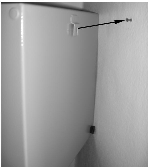
If the controller doesn't seem to fit firmly on the screw, take it down, tighten the screw a bit more and try again. Repeat until the controller seems stable on the screw.
